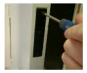
Using the measurements displayed at the start of this guide, mark and cut out the cavity for the Catch Plate in the door at the height required and fit into place using the supplied screws.
