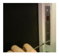
Screw the face plate firmly into the door frame through the screw holes at the top and bottom of the plate.
